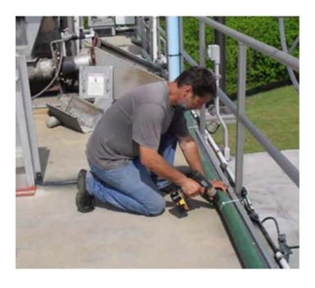
Secure Hose with zipties and drill 10 holes 1/4" diameter facing the odor source. Up to a maximum of 100 feet.
